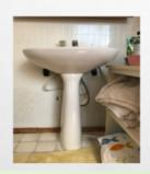
Pedestal sink not properly secured to the wall. Client fearful of holding onto the sink.
